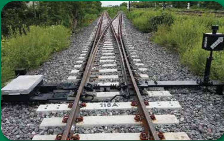
SWITCHING DEVICE – POINT
